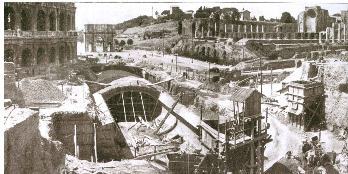
Fig. 2. During the construction of the Line B
