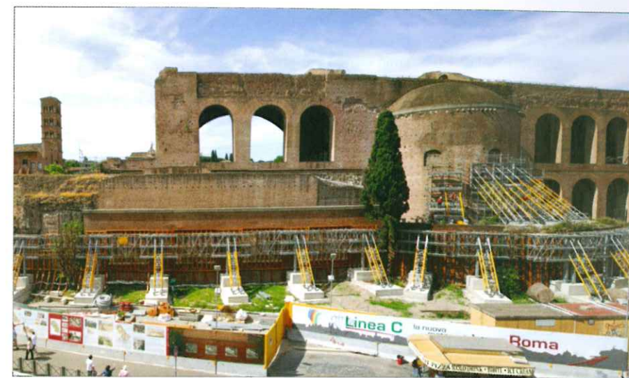
Fig. 5. The reinforcement of Basilica of Maxentius
